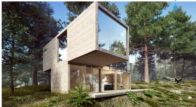
FRONT VIEW CONTAINER HOUSE INSPIRATION
